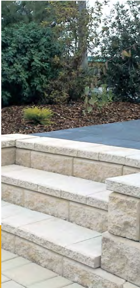
Steps using Allan Block™
