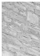
fig. 6. Overgrout Joint
